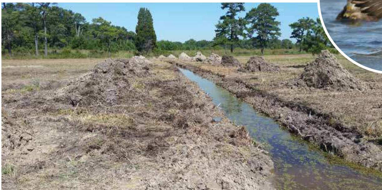
When constructing a wetland, ditches are employed to manage water onsite so that earth can be moved.
